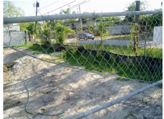
Silt Fence @ Property Line
