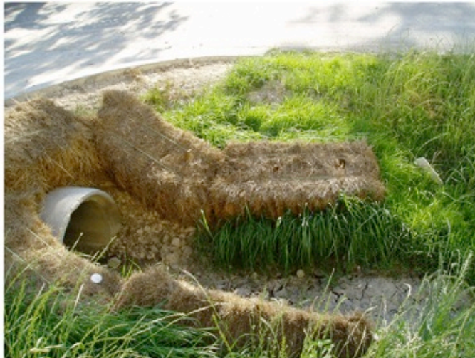
Hay Bales @ Drainage Ditch
