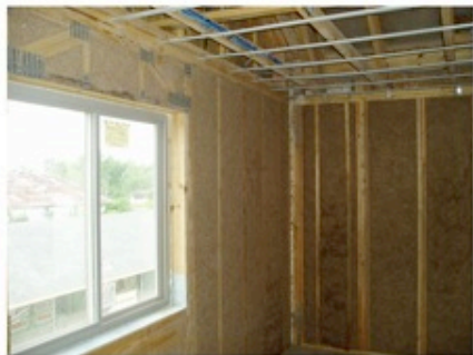
INSULATION Sprayed “CELBAR”
