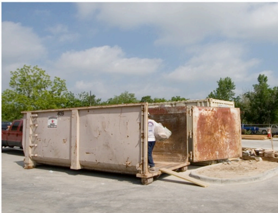
Dumpsters for Off-site Waste Separation
